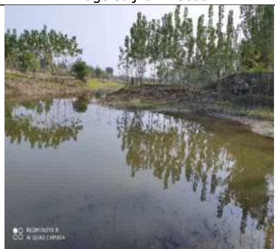
Nahal (Canal Channel) near Sindhauli bridge before C/f with river Pilakhar
