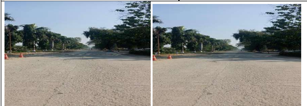
Pic 9 : Paved surface near plantation
