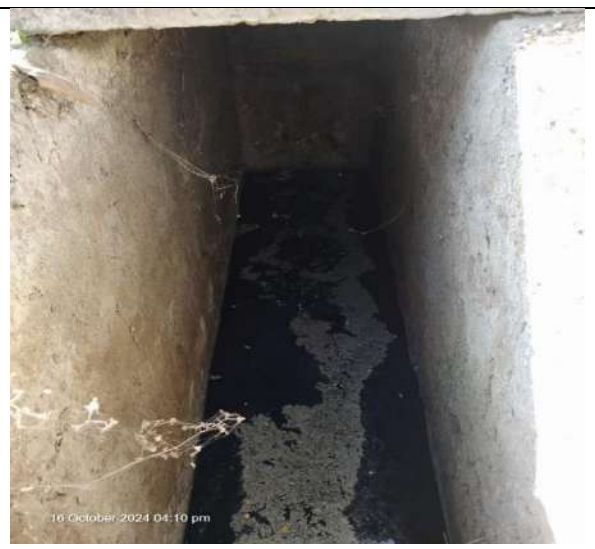
Fig 12: Connecting line with old pumping station blocked
