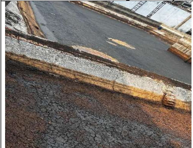
Pic: 7 Sludge and spent wash found stored in settling tank of capacity 2500m3
