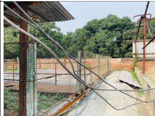
Fig 13: Freshwater line to ETP dismantled
