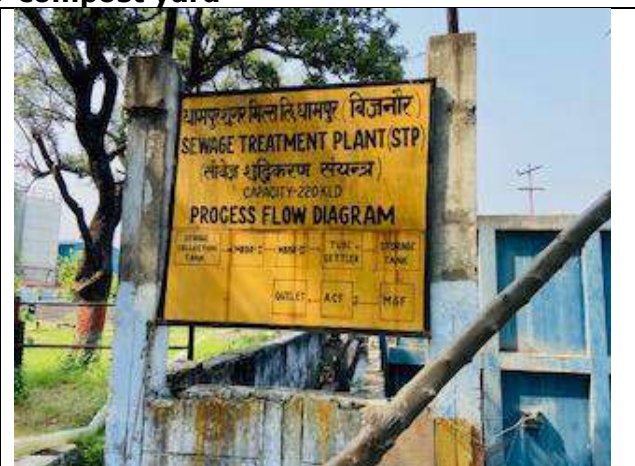
Pic: 5 Sewage Treatment Plant
