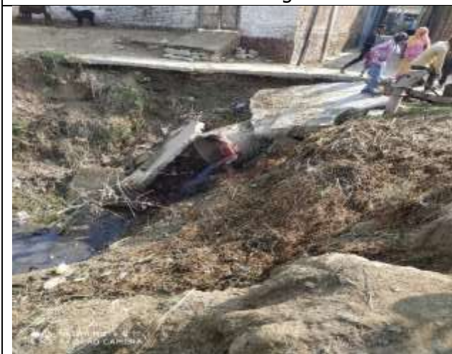
Drain from Sindhauli village near Sindhauli bridge and Chaukidar house
