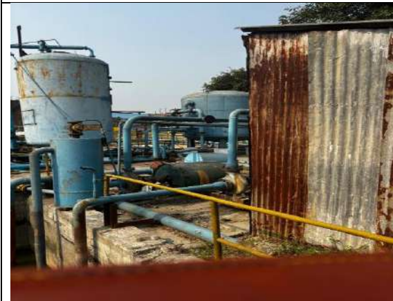
Pic 5: Dismantled the pumping arrangement
