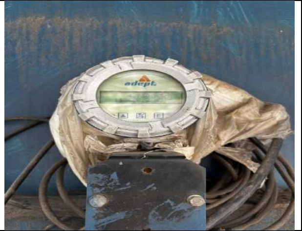
Fig 14: STP inlet flowmeter
