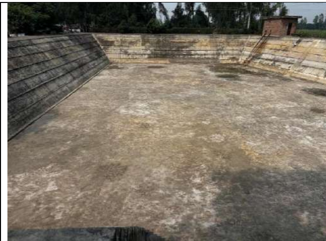
Fig 1: 10000 m 3 brick-lined lagoon
