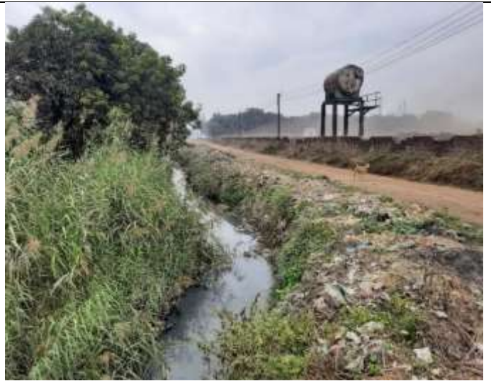
Ikra drain near compost yard of Dhampur Sugar Mill
