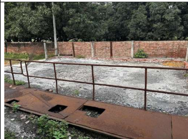
Fig 3: Dismantled old pumping station
