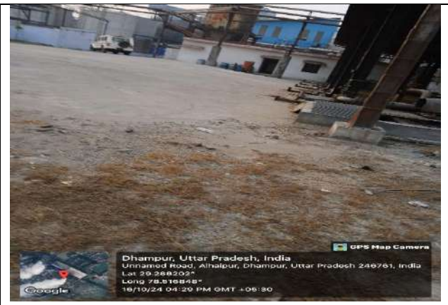
Pic:2 Dismantled 3 rd borewell and concrete the area with cement
